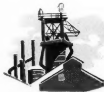
THE HANNA FURNACE CORP. Buffalo, New York. Blast furnace division for production of various types of pig iron.
